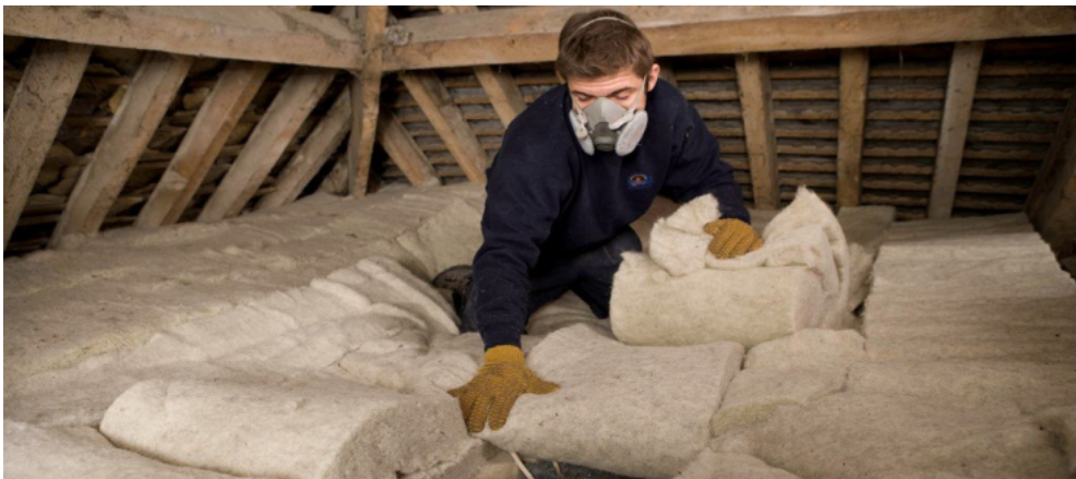
Cold roof insulation at ceiling joist level
