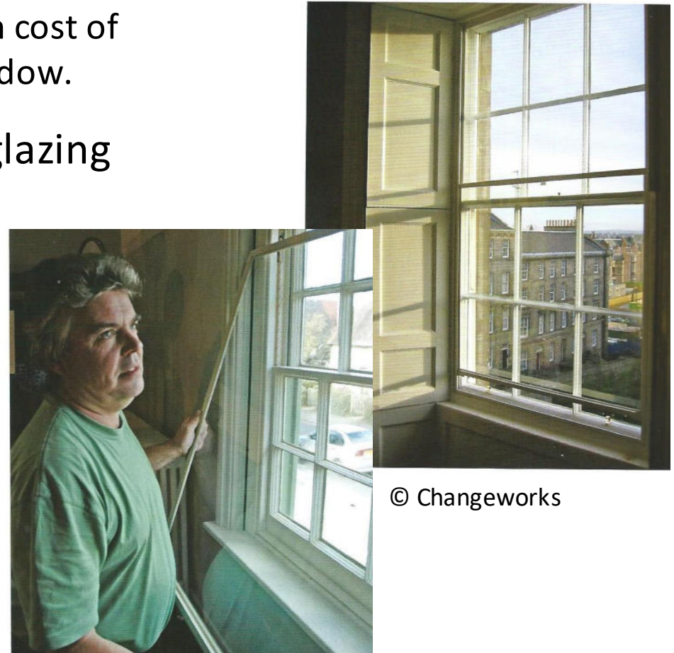
Installing secondary glazing © SPAB
