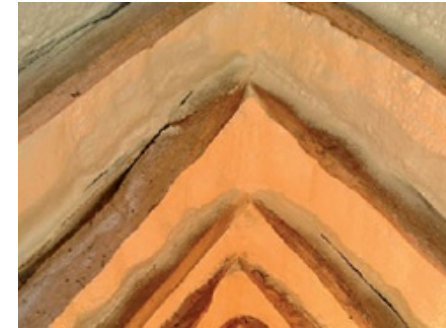
Blown foam insulation
